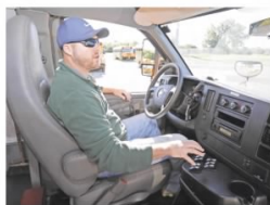
Rick Bogart of Kobussen activates the safety lights on a switch panel inside a bus.
